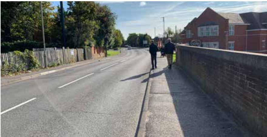
Photo.15 View east from railway bridge crossing
