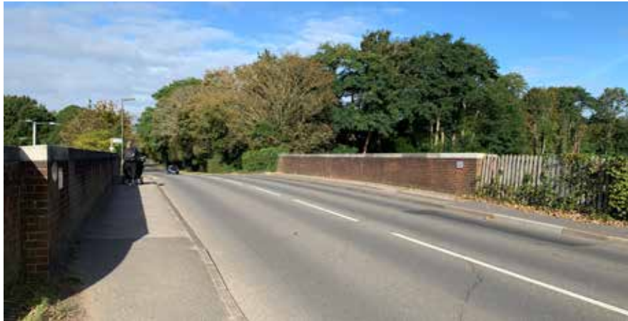
Photo.09 View west towards station access
