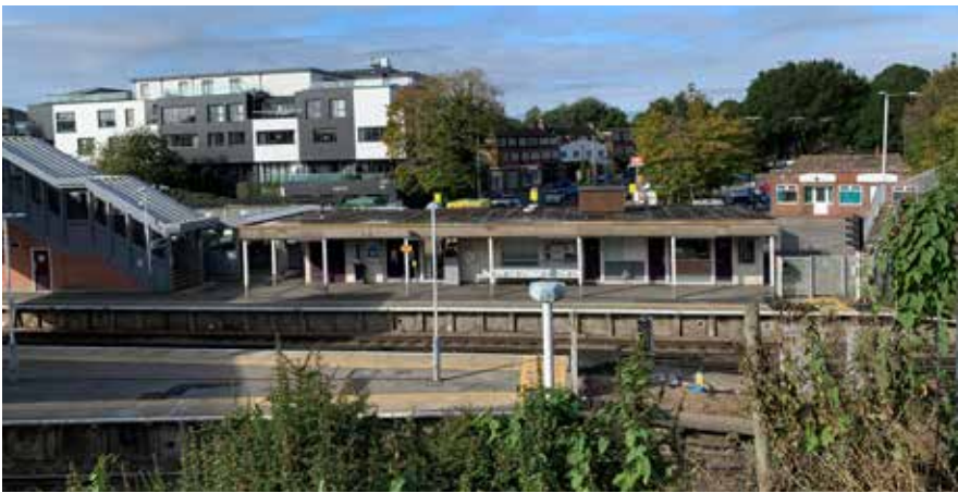
Photo.17 View to station from Christchurch Road
